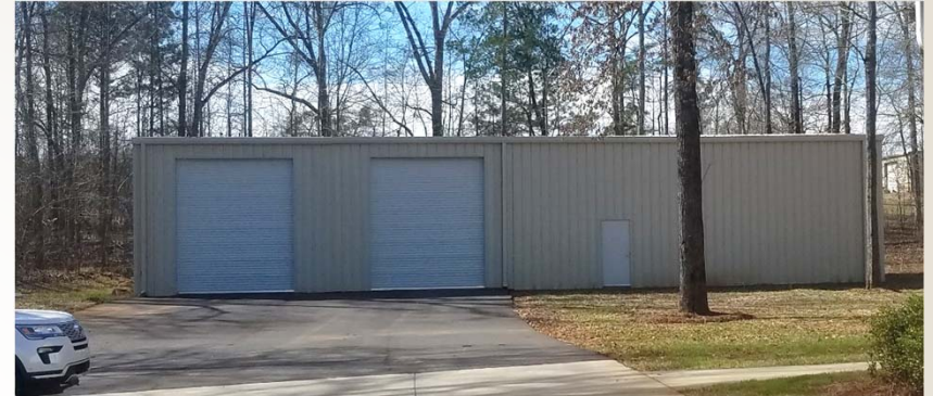
4,000 SF Warehouse Building
